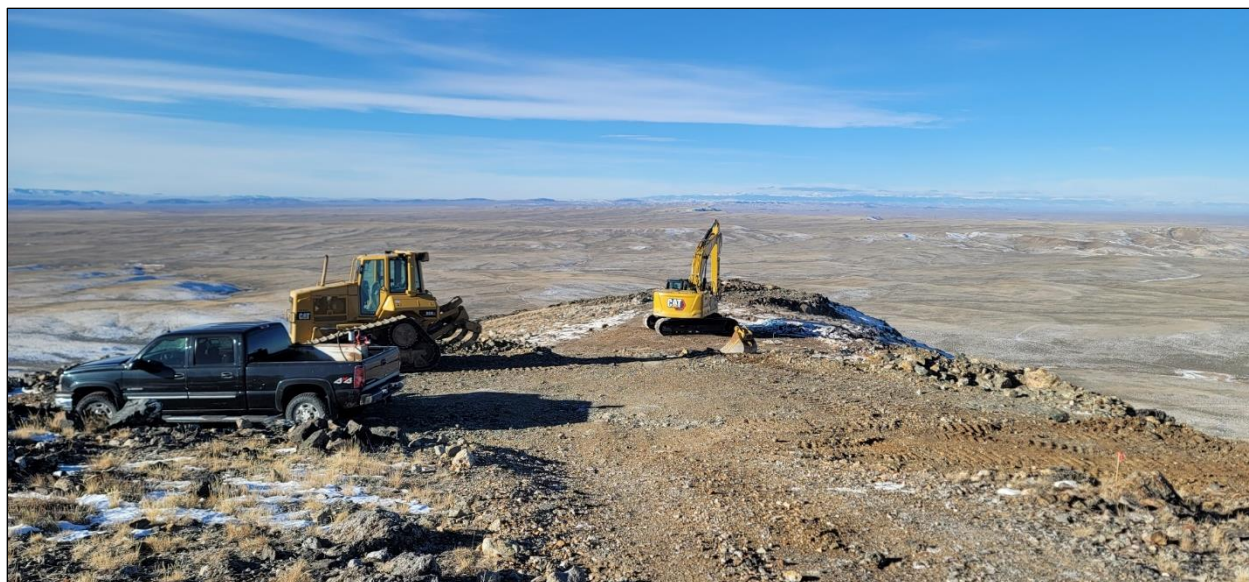
Figure 2: Road and Drill Pad Construction at Black Mountain
